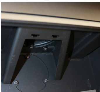
4. Removal of the baffle gives immediate access to the flue for sweeping and maintenance.
